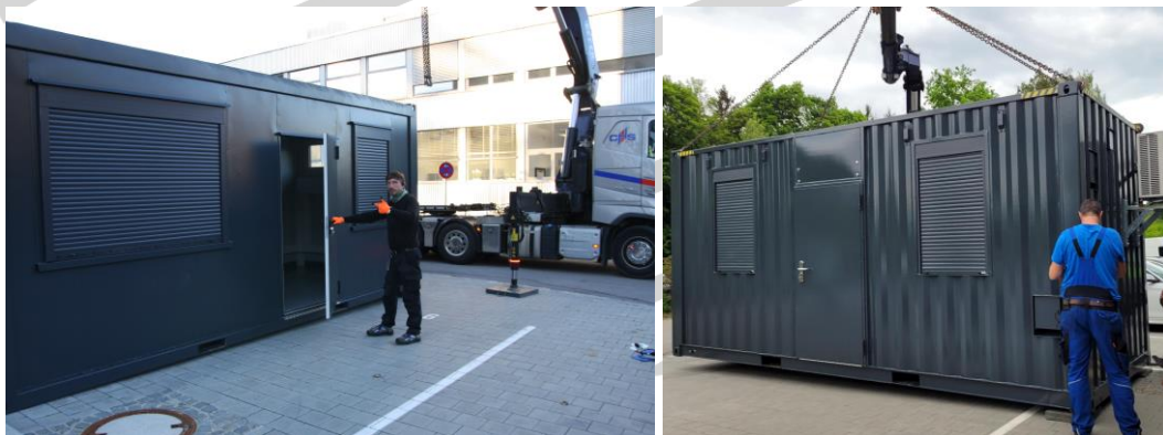
Figure 2: Delivery of the two J.A.M.E.S LabContainers (spatial element and ship container type)
